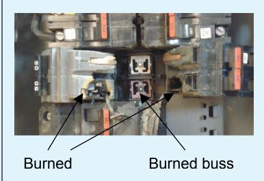
Authorities recommend that an immediate professional inspection be done because Federal Pacific Electric panels cannot be counted on to always protect homes from overcurrents or short circuits that could result in a fire.
